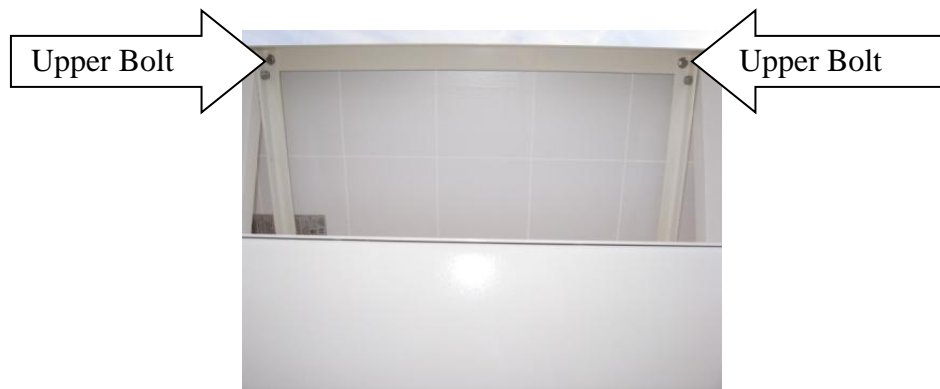
Figure 10. Upper Solar Panel Mounting Bolts
