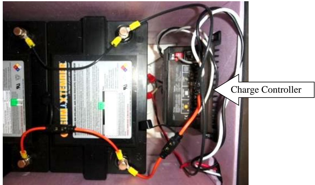
Figure 6. Battery Installation
