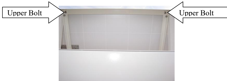
Figure 10. Upper Solar Panel Mounting Bolts
