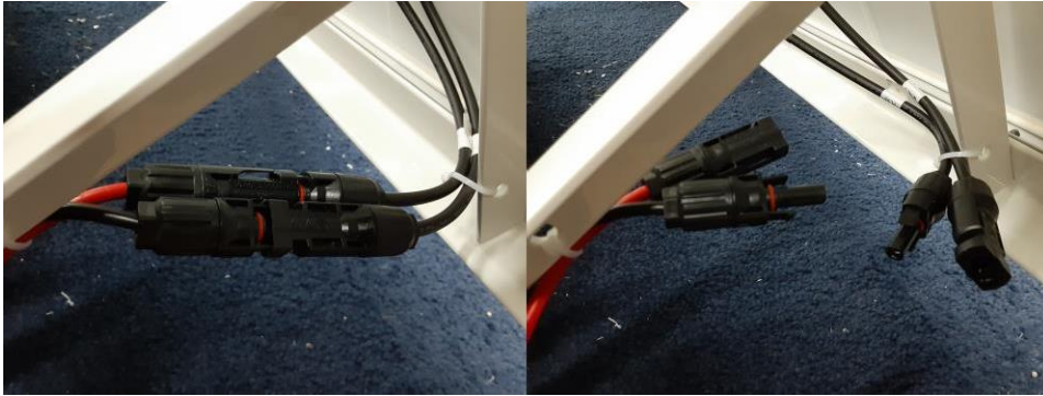
Figure 8. Solar Panel Connectors
